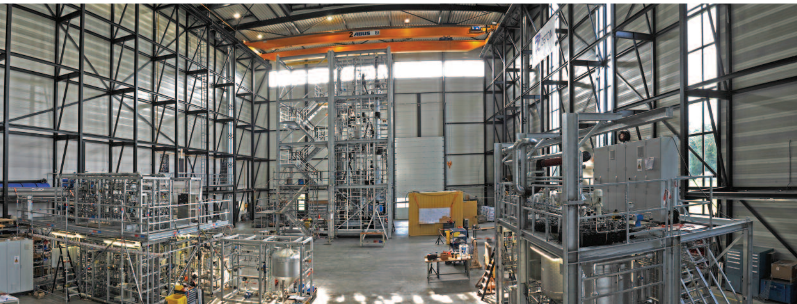
Overview of the high bay for construction of modular pilot plants.
